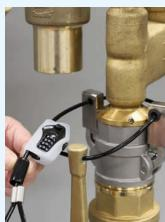
Shut off the MODU lower section and remove the MODU supply head by opening the camlock coupling.
