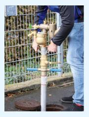
Attach the standpipe security device.
