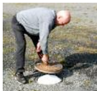
4. Do not forget to put in the insulation cushion before closing the cover.
