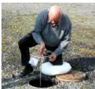
1. After removing the cover and insulation seal, take out the meter system, turning the wheel slightly while doing so.
