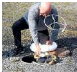
2. The flexible hose allows the meter system to be conveniently placed next to the pit opening and a reading taken or the meter replaced.
