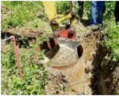
An old pit is replaced
