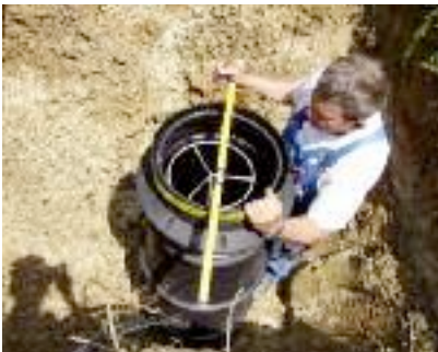
Levelling of the EWE telescopic pit
