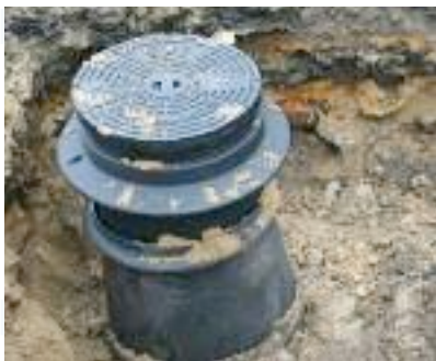
Compaction in layers at installation
